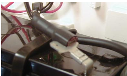
Y-terminal adapter installed on negative battery terminal
